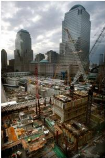
EARLY WORK ON 1 WORLD TRADE CENTER. PHOTO: MARIO TAMA/GETTY IMAGES.
